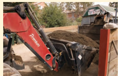
6. Removal of compost to stockpiles
