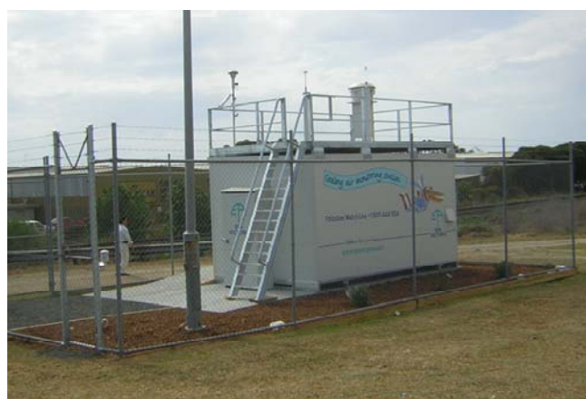
Figure 5: Upgraded monitoring station at Geelong South
